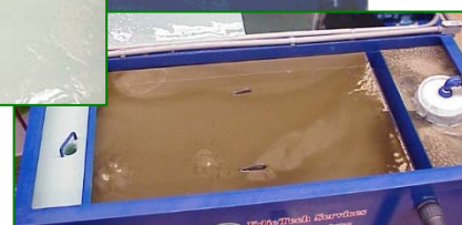
Tramp Oil Removal
